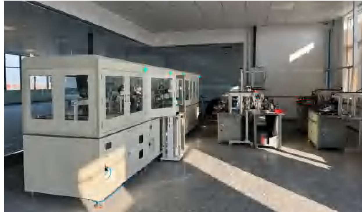
Fully Automatic Current Transformer Assembly Production Lines (2 Lines)
